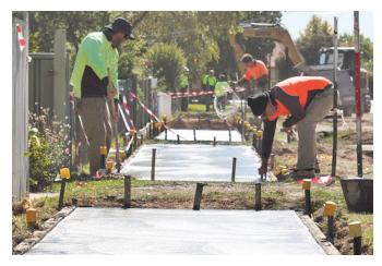
The eastern side of the footpath on Coster Street, from Bridge Street to Samaria Road, is being upgraded and widened as part of the Pathways to the Future program. Works are scheduled for April and will see the footpath widened to 1.5 metres to enable scooter and wheelchair traffic easier access to Benalla Health
