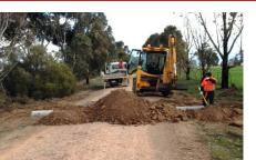
We installed new pipes in Peck Road, Goorambat. This allows drainage under the road, so that water doesn't impact on the quality of the road surface.
