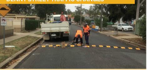
New traffic calming devices (speed humps) have been installed in Denny Street. These devices are speed limited to 10km/h. It is designed to slow traffic down around the Denny Street carpark, making it safer for pedestrians and road traffic.
