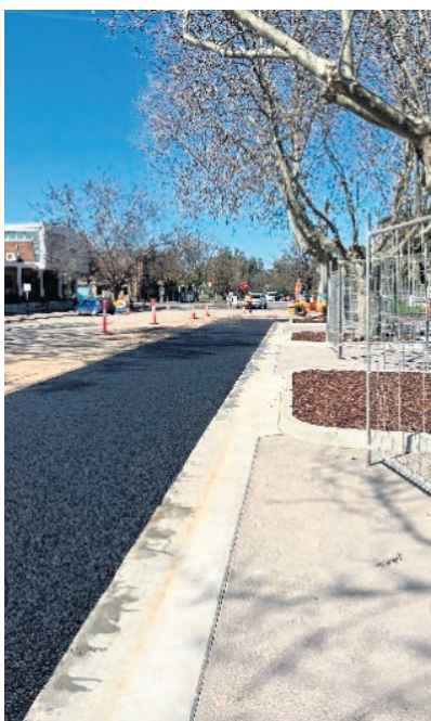
Road surface improvements along Mair Street.
