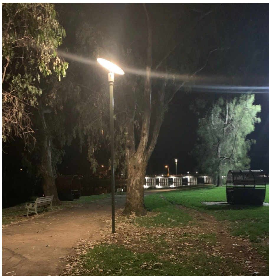
New lights installed on the Lake Benalla Walking Track.
