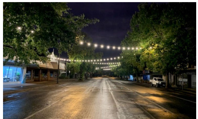
Festoon Lighting at night (Nunn Street, Benalla).
