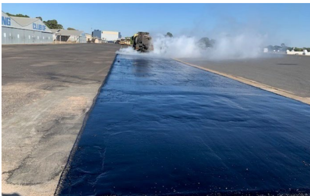
Airport hardstand reseal works underway.
