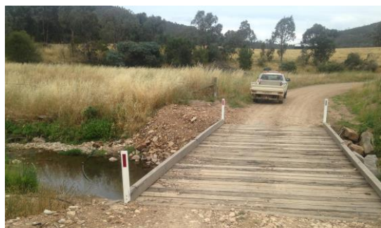
WATCHBOX CREEK ROAD BRIDGE
