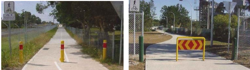
Option 3: Staggered fence treatments slow cyclists but need to be properly delineated.
