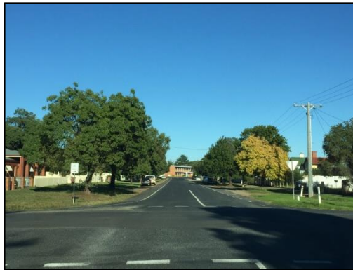
Figure 3.3.10 Wedge Street Bicycle Lanes
