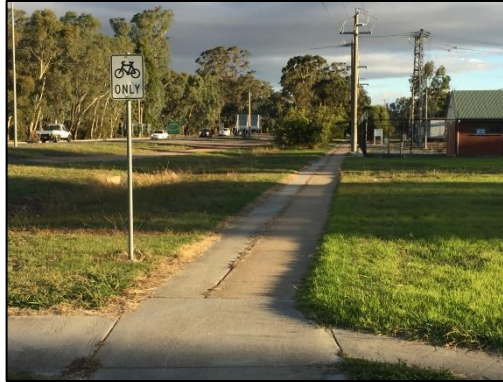
Figure 3.2.1: Mansfield Road Off-Road Bicycle Path
