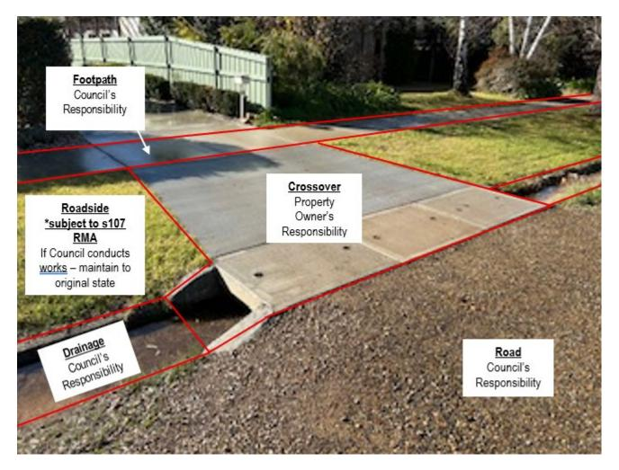
This diagram shows a box culvert/ open drain crossover
